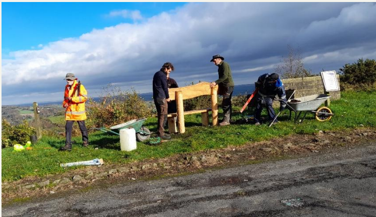
BWE rustic benches being erected at DCC owned picnic site – Highoredish. Richard Felton (the instigator!) is inspecting the work, credit Karen Haywood, 3 November 2023
